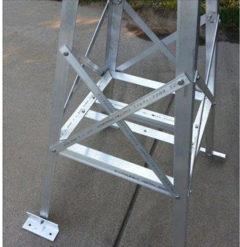
6. When all X-braces and shelves have been installed, tighten all hardware securely with a wrench.
