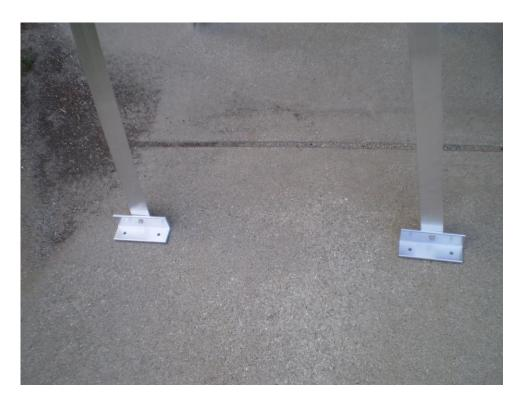
9. Make sure that the tower is on a level surface. Place a level across the top of the thrust bearing, then tighten the 8 bolts that hold the top angle brackets to the 4 legs. There will be a small gap between the legs and the top brackets even when tight. Make sure that the thrust bearing AND rotor shelves are both level in 2 orthogonal directions. Securely tighten the remainder of the hardware at this time except for the bolts that hold the feet.
