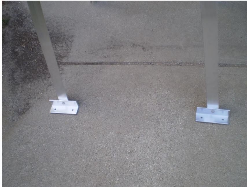
11. Make sure that the tower is on a level surface. Place a level across the top of the thrust bearing, then tighten the 8 bolts that hold the top angle brackets to the 4 legs. There will be a small gap between the legs and the top brackets even when tight. Make sure that the thrust bearing AND rotor shelves are both level in 2 orthogonal directions. Securely tighten the remainder of the hardware at this time except for the bolts that hold the feet.
